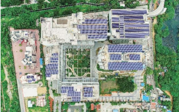
Fig. 4.7: Rooftop Solar at IITMRP
