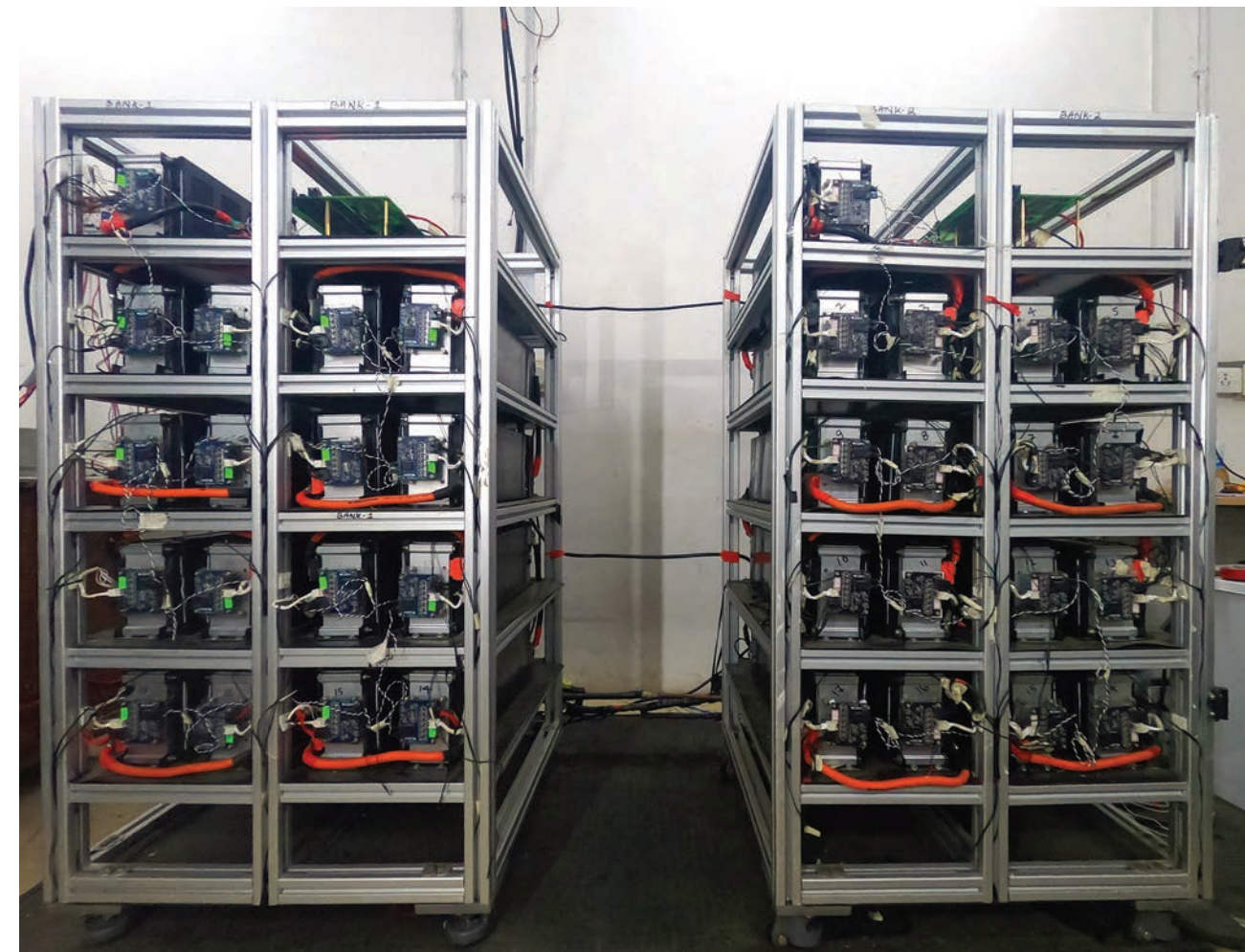
IITM Research Park’s lithium-ion battery facility stores excess electricity for use after the sun goes down or when there’s a dip in wind power.
